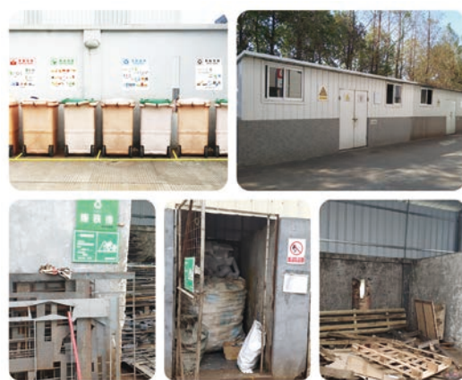
The plants set up storage areas and warehouses for different types of wastes to prevent recyclable wastes from being mistakenly treated as non-recyclable wastes
